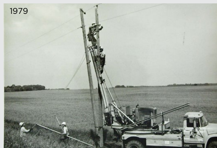
REA crews replacing a pole using a pressure digger truck. The Co-op spent $48,000 on this truck in 1974.
