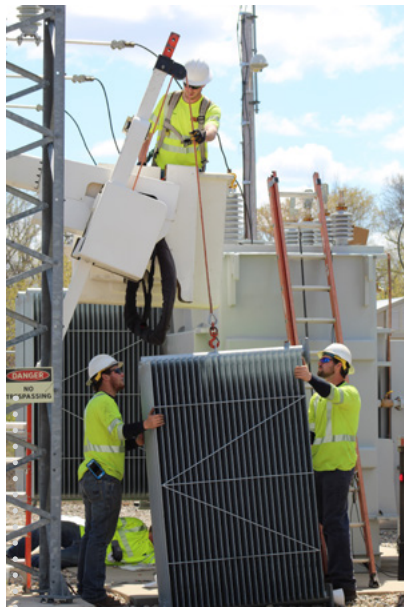
REA Linemen install a new radiator for cooling the transformer oil at the Leaf Valley Substation.
