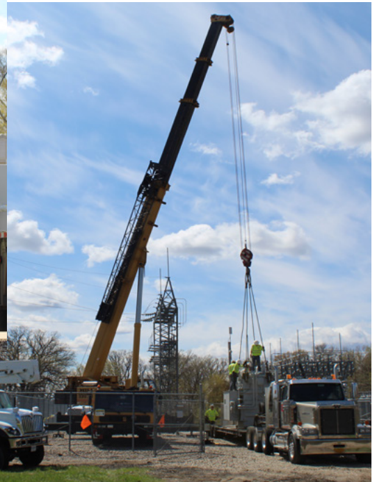
A crane removes the old transformer and places the new transformer into the Leaf Valley Substation located north of Garfield.
