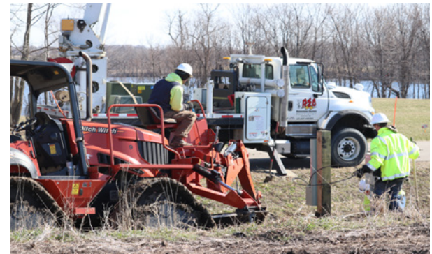
REA crews install a new service on the south side of Turtle Lake.
