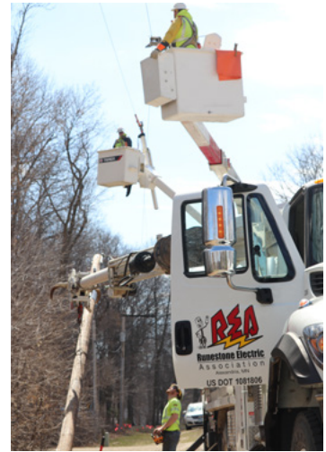
This spring, REA crews have been busy maintaining the system by replacing power poles and plowing underground. This photo was taken on the northeast side of Lake Miliona.
