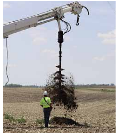
Lineman Troy Pederson augers the hole in preparation for the new pole installation
