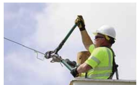
Lineman Joe Friedrich crimps the bail to the phase wire
