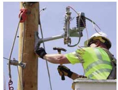
Lineman Joe Friedrich drives a lag into the crows foot
