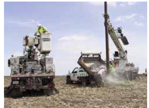
Linemen Troy Pederson and Luke Gilbertson fill the hole surrounding the new pole with rock
