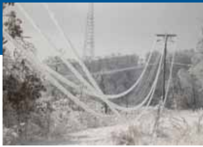
Ice and frost on powerlines can lead to flickering and blinking lights.
